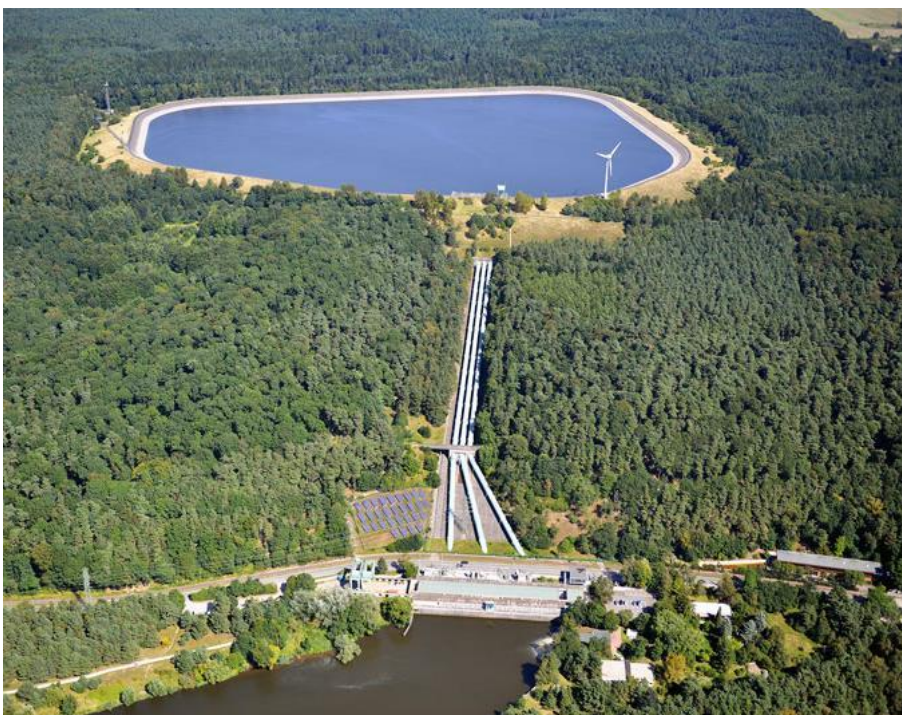
Figure 10 The Geesthacht pumped hydro storage plant in Germany. Photo credit: Vattenfall AB
